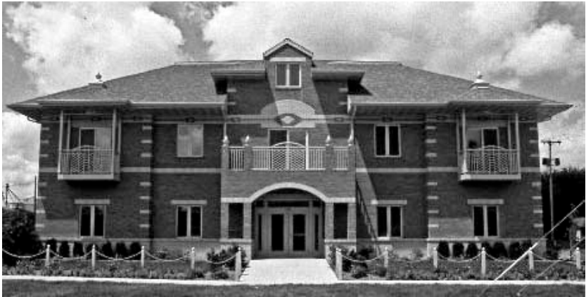
Maharishi Sthapatya Veda office building, Fairfield, Iowa, U.S.A. 146
