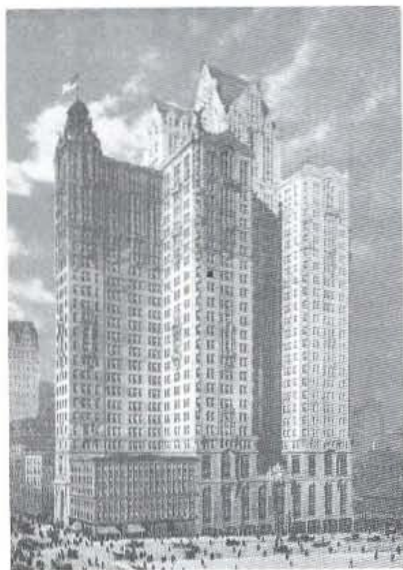
Benenson (City Investing) Building, 1908 (Francis H. Kimball, architect). Irregular plot extruded to a height of 480 feet, "13 acres of floor space, and room for 6,000 tenants..."
