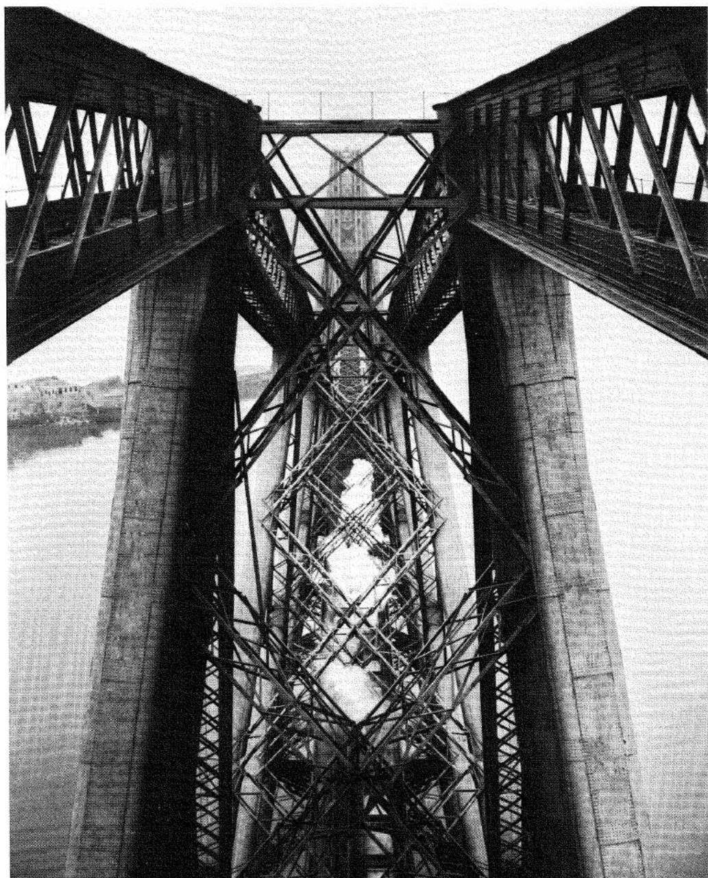
6. The Forth Bridge, view S. from top of N. pier.
