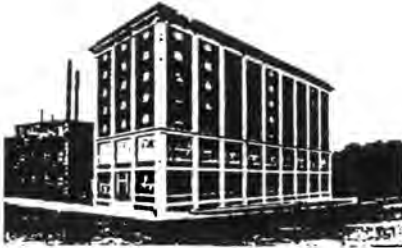
Paramount Knitting Co., Kankakee, Ill. Combined warehouse and manufacturing space. Built 1914
