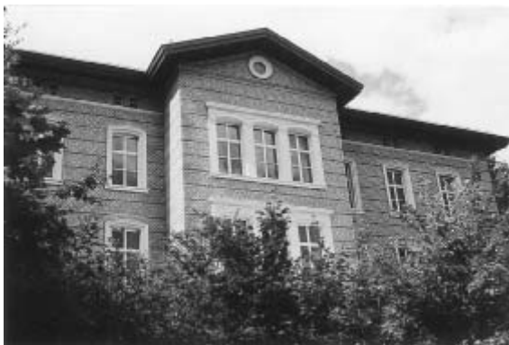
13.6 Landeslinik Eberswalde . Building designed by Martin Gropius in 1865. Photograph by J. P. Boudreau, 2000.
