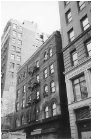
10.3 228 West Eighteenth Street, New York City. Photograph by J. P. Boudreau.
