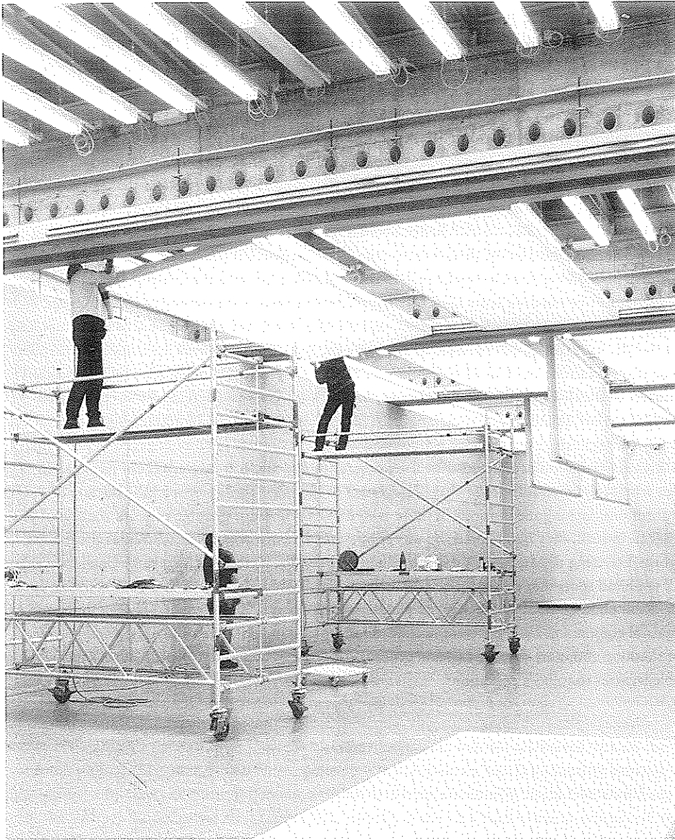
The making of, Generali Foundation (1998), dismantling of ceiling panels during installation
